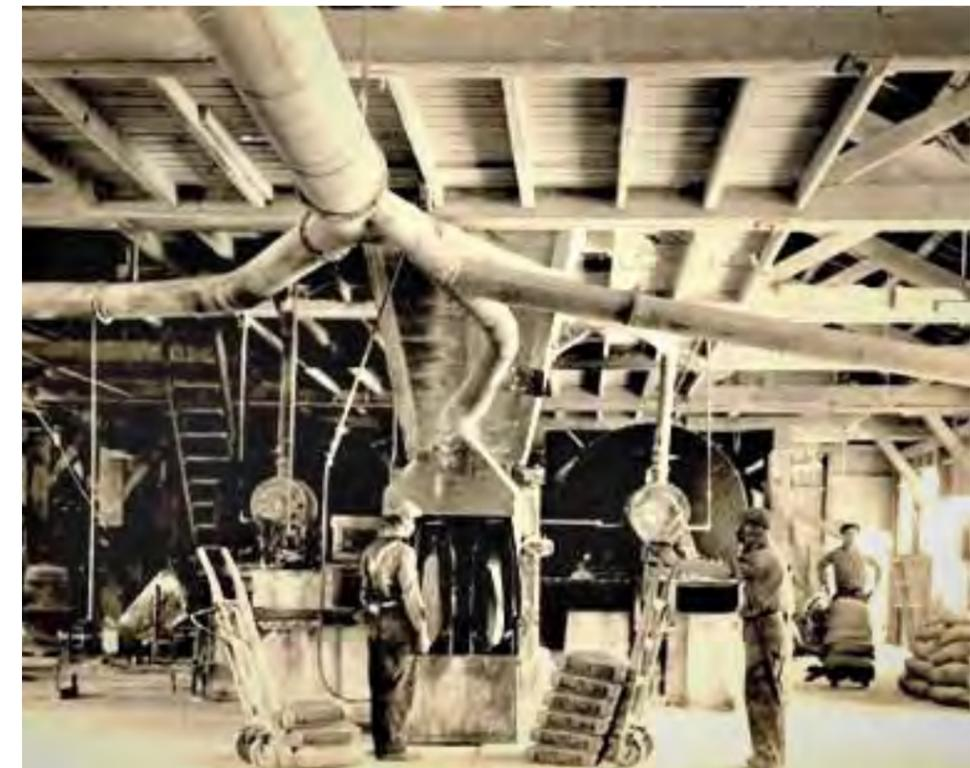
*Pulverizing plant interior c. 1930s with sorting and packing equipment. For over 50 years, all finished products left the site via rail. (Courtesy, Al Stokely)*
