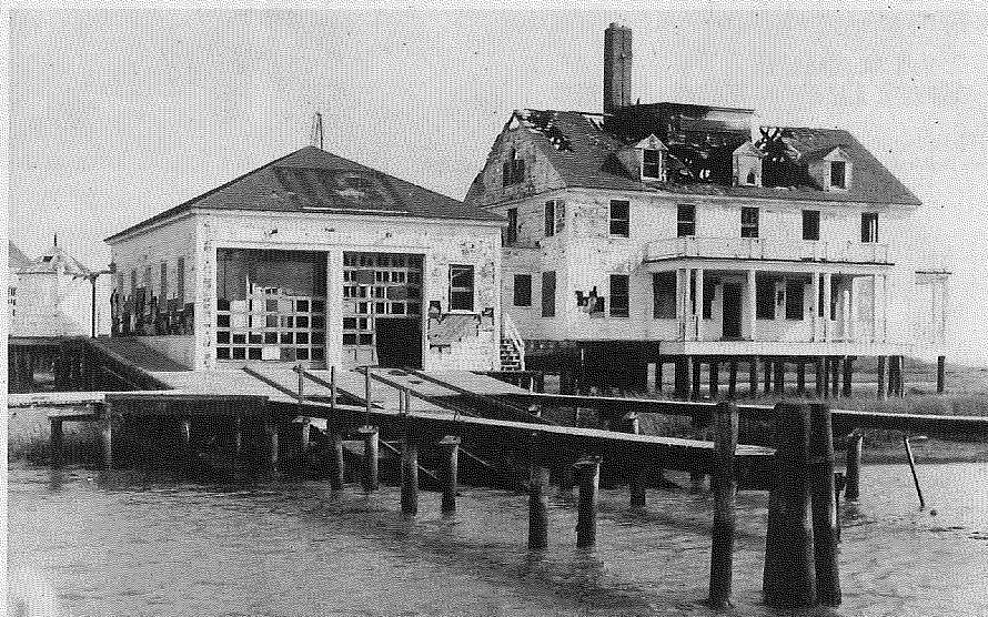
Fig. B – After the fire with roof burnt off.
