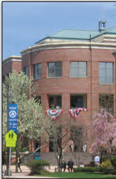
Planning, Engineering, & Roads Annex, Toms River, NJ
