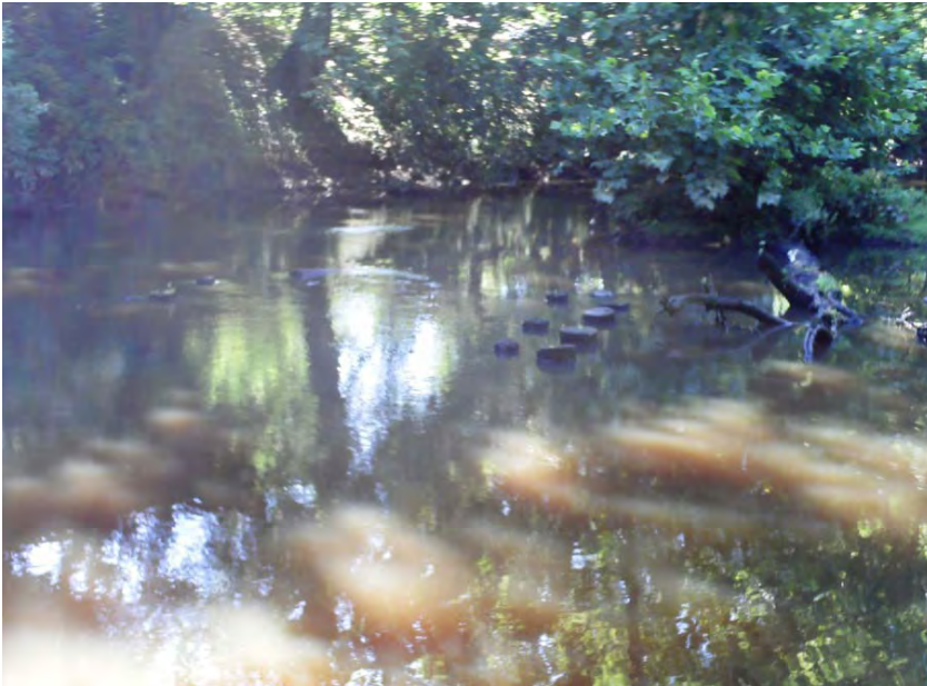
Figure 9: The Crosswicks Creek is shown here at the point where the timber rail bridge once spanned it. The pile stumps can be seen just above the water line. The required span is estimated to be 86 feet.
