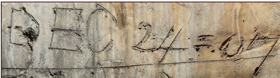
Plaster graffiti found on chimney. Photo credit: C&H Staff
