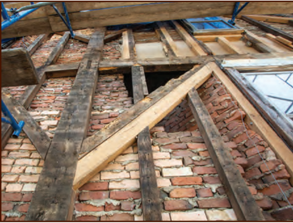
Exterior framing repair, West Wall
