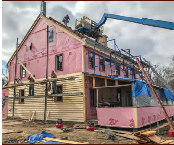
Yellow Cedar being installed.
