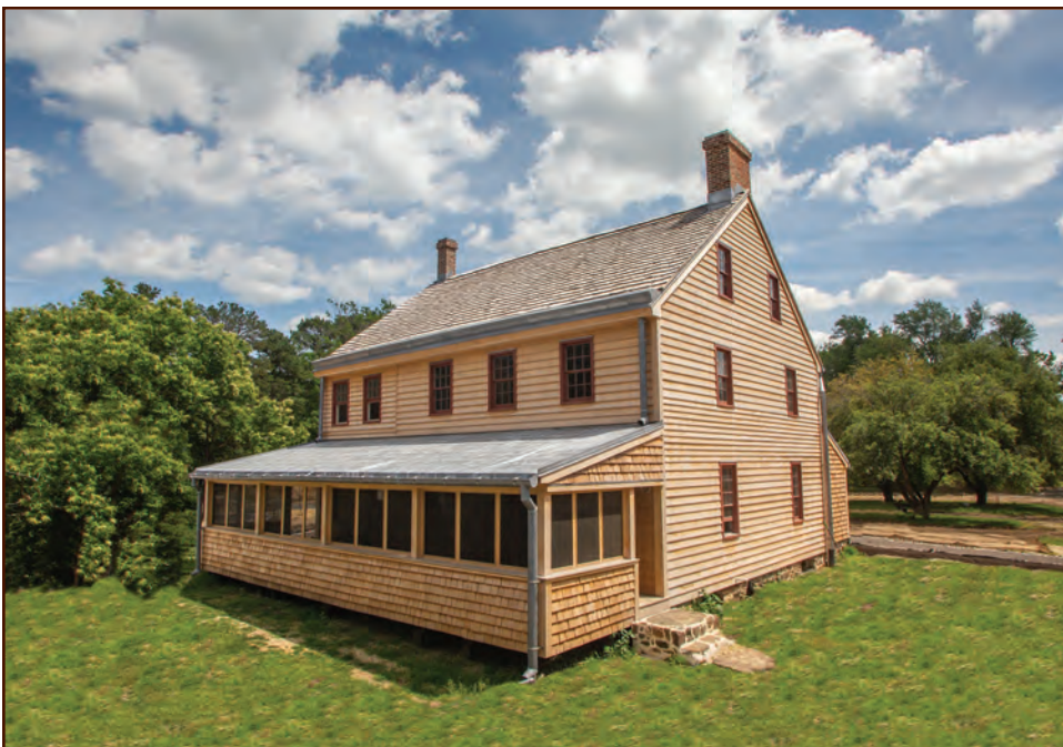
Cedar Bridge Tavern Completed Photo credit: Ocean County Department of Parks & Recreation
