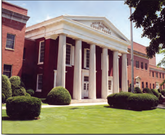
Courthouse and West and East Wings sometime after 1950
