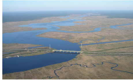
Fig. 2. Aerial photo of Mullica River where it is crossed by the Garden State Parkway
