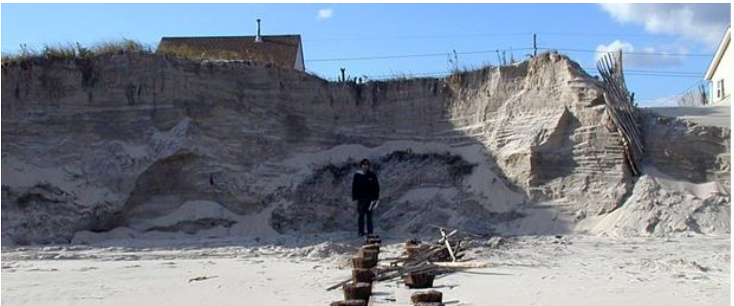
Figure 4.1-1 Heavy erosion displayed at beach in Holgate, NJ (CRC, 2007)
