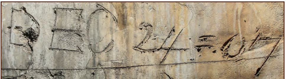
Plaster graffiti found on chimney. Photo credit: C&H Staff
