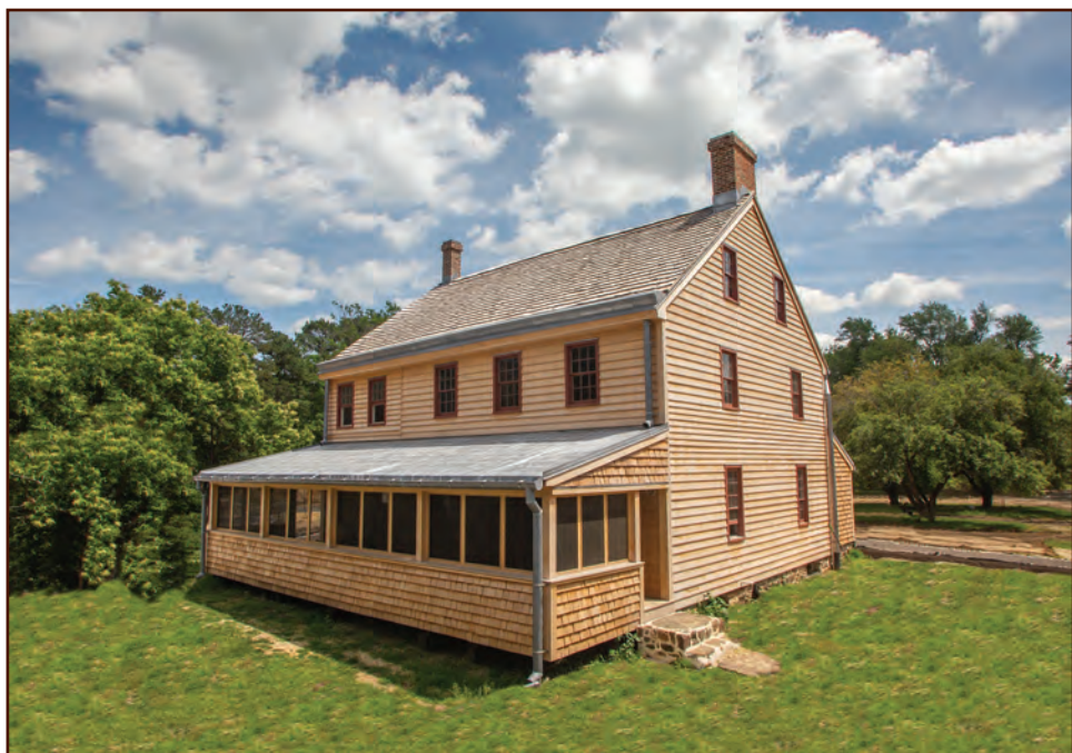
Cedar Bridge Tavern Completed
