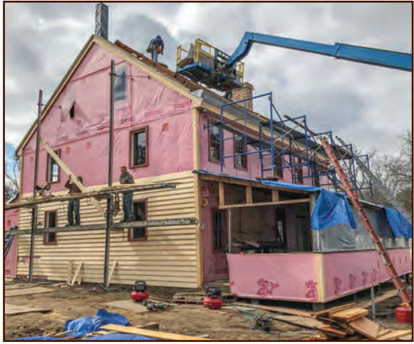
Yellow Cedar being installed.
