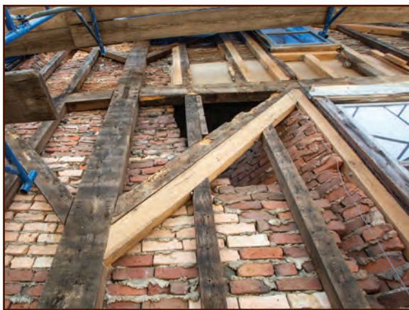
Exterior framing repair, West Wall
