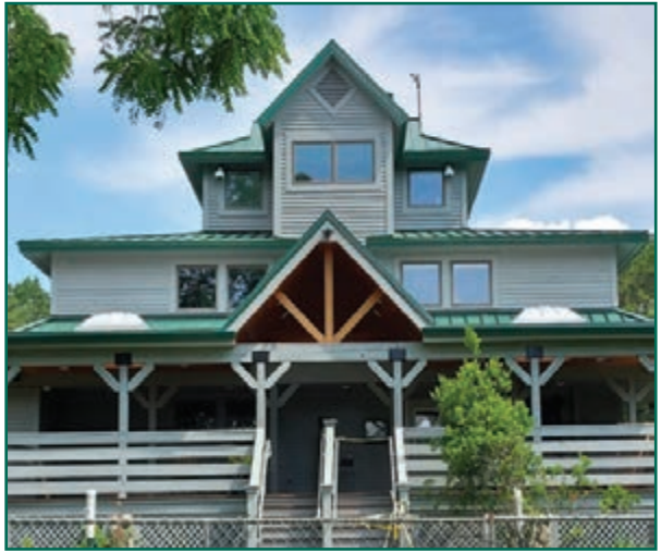
Updates underway at Wells Mills County Park. Photo Credit: Pat Johnson
